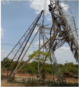
Fig: 4. Crematorium tracking stand aligned with back crane and reflector frame
